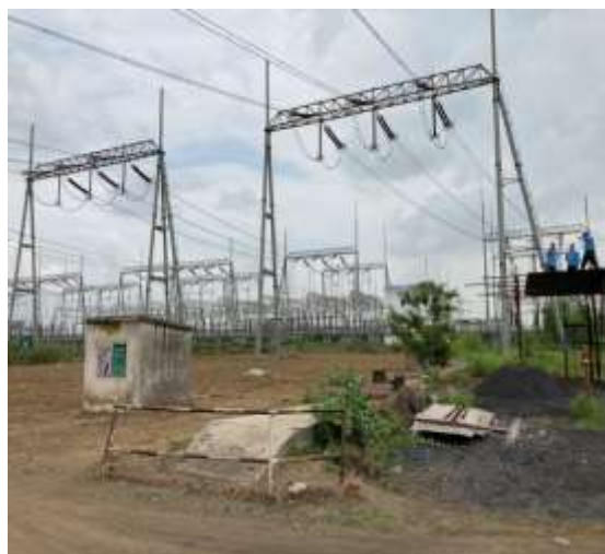
GT Transformer Gantry Tower and Switchyard
