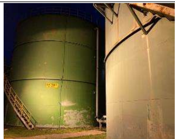
4X1600M3 Capacity DM Tanks
